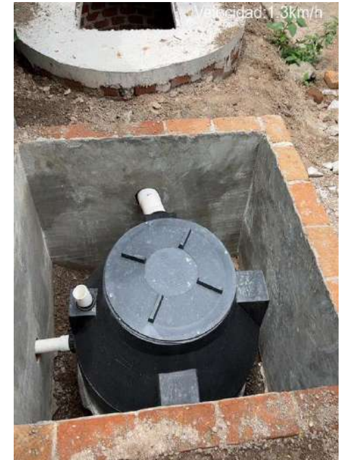
BIODIGESTOR INSTALADO
